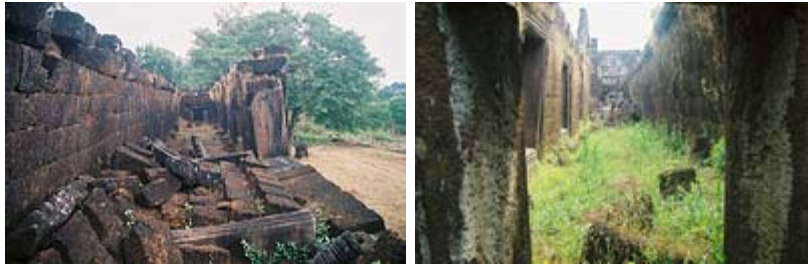
Corridors looking East and South in Northern Palace
