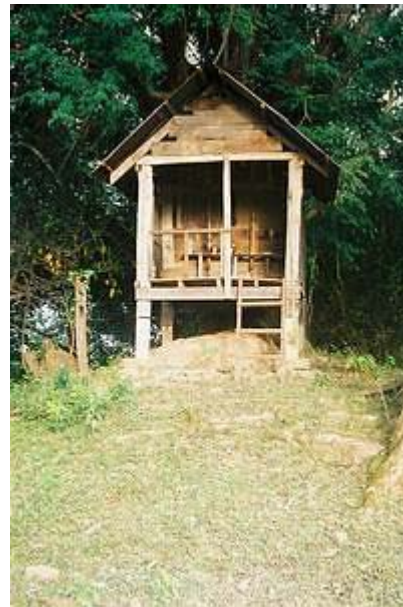
Shrine after restoration
