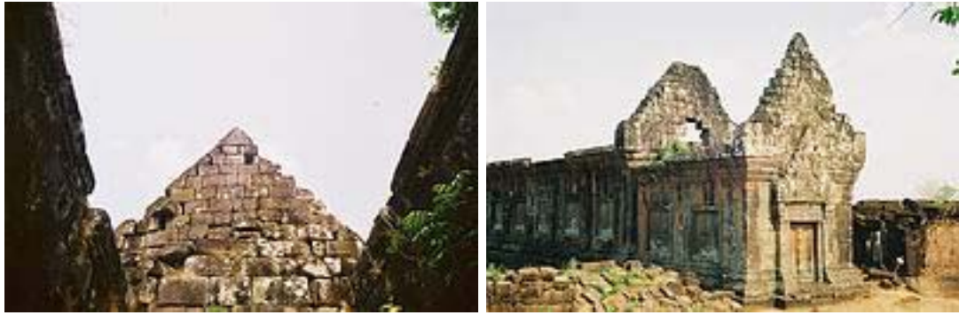
Double Tiered Roof of Southern palace looking West and SE
